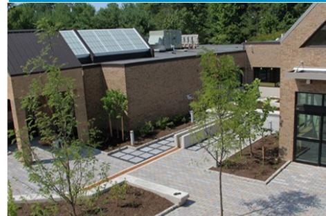
Permeable pavers allow rainwater to enter the ground. Photo credit: BioHabitats
