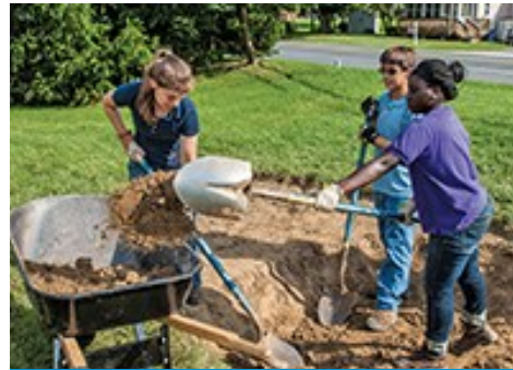
The raingarden under construction
