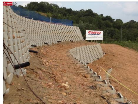
The retaining wall being installed in steep, non-porous clay earth site. Photo Credit: BUBBA Awards
