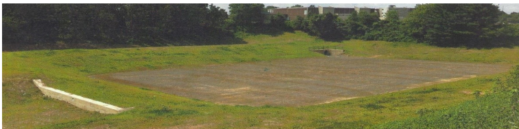
The new surface sand filter:
