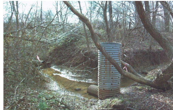
BEFORE: The former creek bed with sediment trap.
